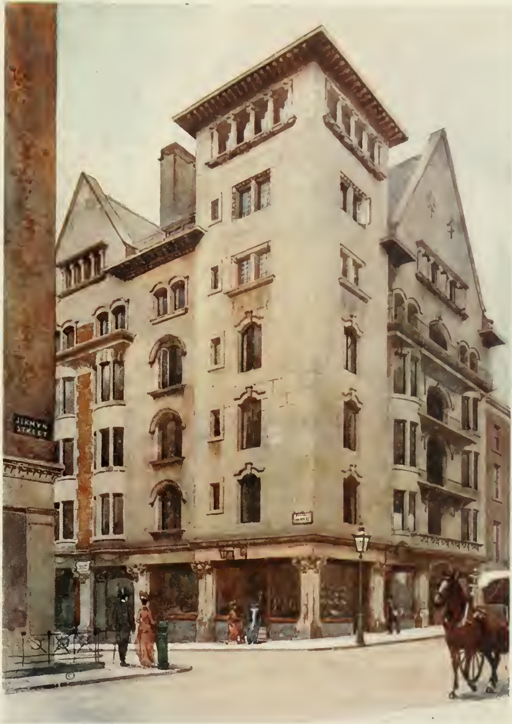
MARLBOROUGH CHAMBERS, JERMYN STREET, LONDON, W. FROM A DRAWING BY F. HAMILTON CRAWFORD. THE BUILDING IS FACED WITH PORTLAND STONE AND BACKED WITH BRICKS. THE HEIGHT FROM THE GROUND FLOOR TO THE TOP STOREY IS 54 FEET. FROM THE GROUND LEVEL TO THE CORNER OF THE TURRET, 71 FEET; AND TO THE TOP OF THE GABLE, 86 FEET.
